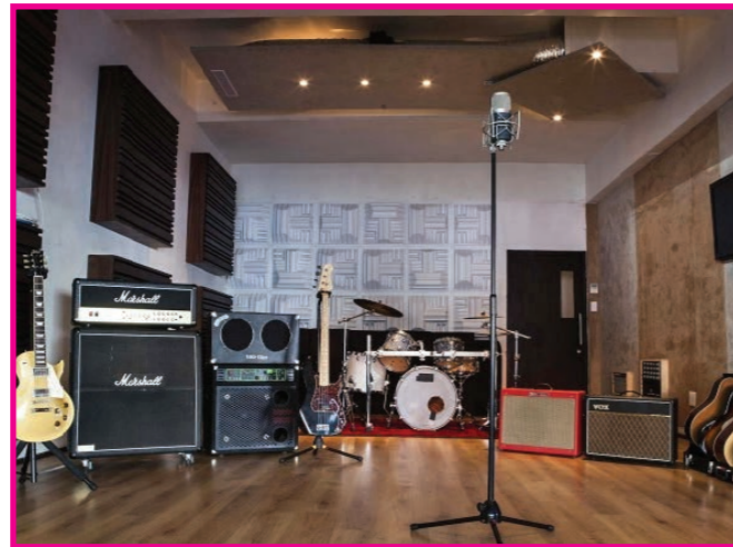
Diffusers and absorption panels
