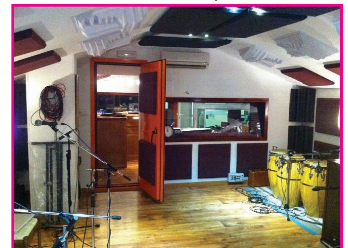
Acoustic panels and diffusers
